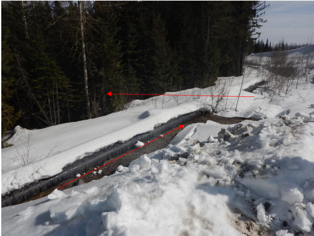
Figure 13 March 29, 2023. Path of flow from sump along pipeline and into adjacent forest.
