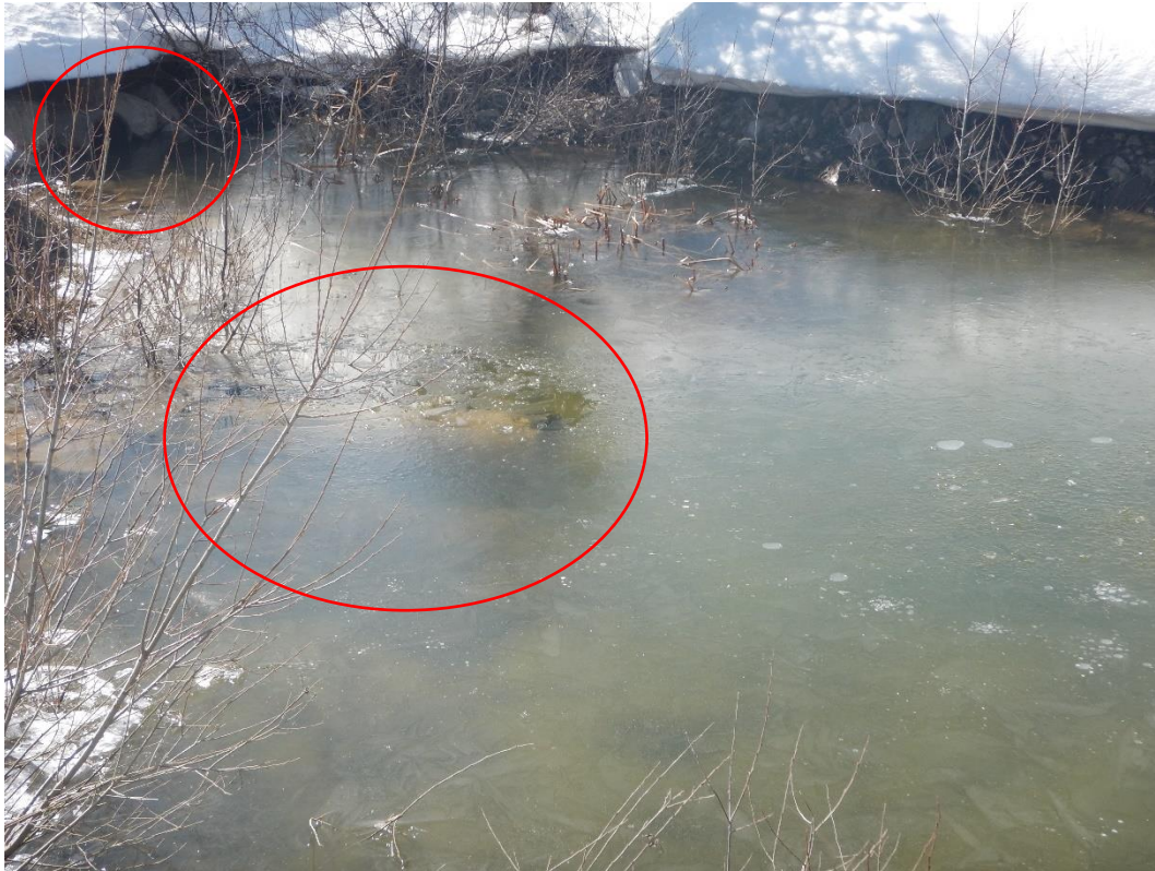
Figure 10 March 29, 2023. Upper Long Ditch Sump with primary pipeline submerged. The pipeline is frozen and not conveying water. Discharge to Lower Long Ditch Sump in upper left.
