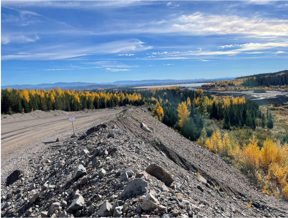
Photo 3: View Southwest to the Southern Portion of the Proposed Rock Disposal Area, with the Existing Tailings Pond in Background. Bootjack Creek Follows the Green Deciduous Tree Stand in Middle of the Photo
