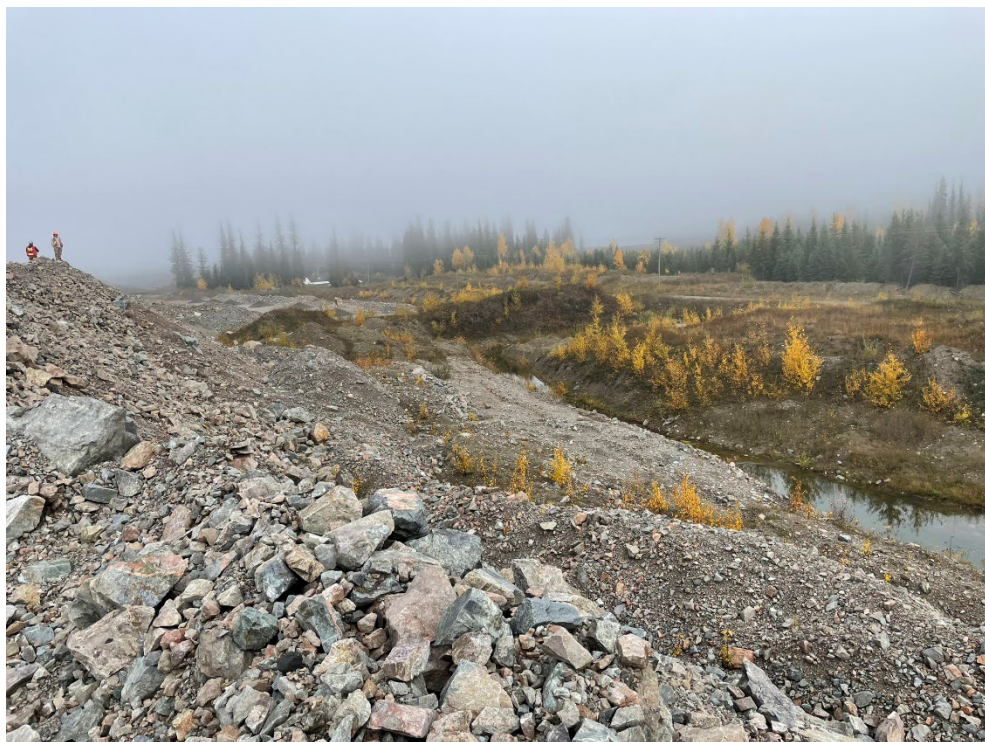
Photo 6: View Northwest Through Northeast TSF Foundation Preparation Area
